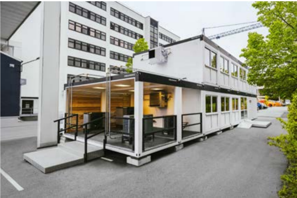
Two heat pump modules were installed in two ELA terrace containers with open sides for training purposes.
