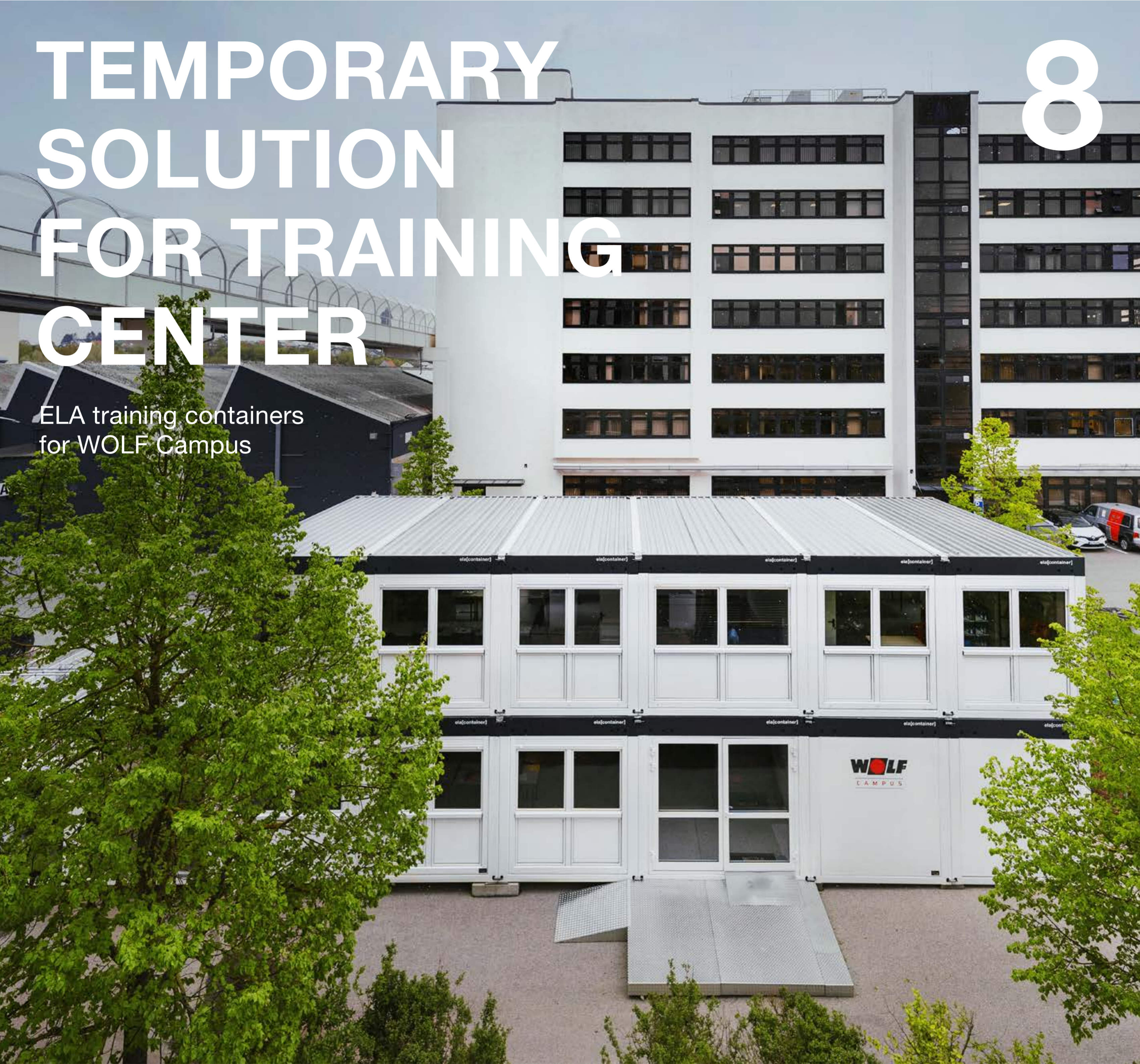
The temporary training center for WOLF consists of 14 ELA training containers, providing around 220m² of usable space in total across two floors.
